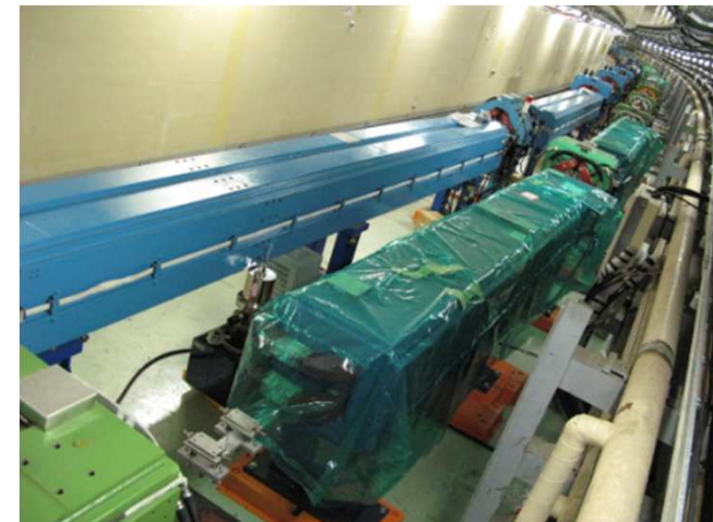
100 new bending pipes are installed
