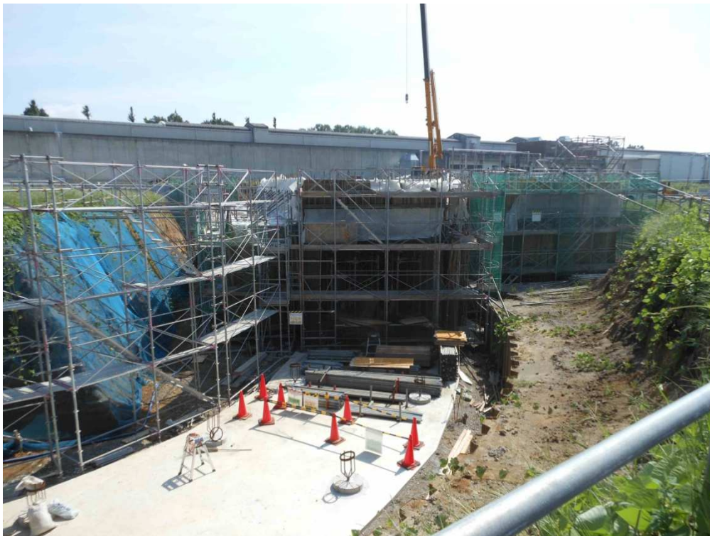
Tunnel construction for new bending ring
